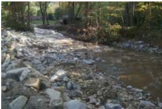
Same creek reach looking downstream following some bank repair work.
