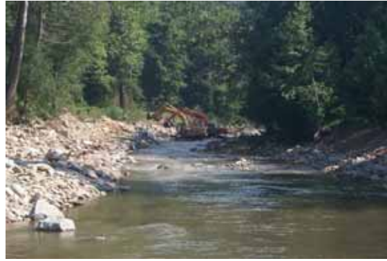
EWP stream repairs underway on a NC trout stream.
