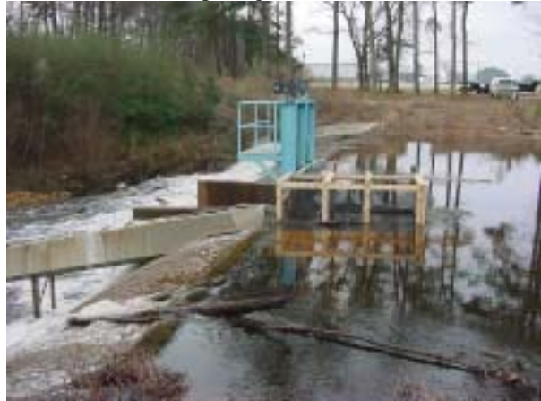
Holts Lake dam fishway.
