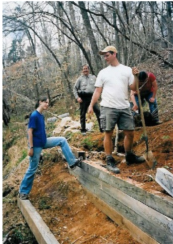
Lori Davias and Edward Malindzak stop to admire their work. Several students built a retaining wall and planted trees along the Eno River to stabilize the bank.
