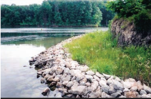
By adding native plants to riprapped shoreline, erosion is controlled and the aquatic habitat is enhanced.
