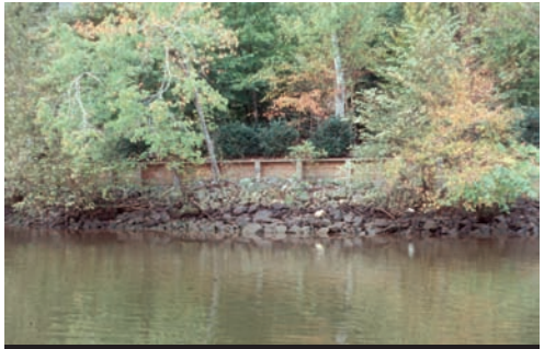
By adding riprap and native plants to a seawall, the fish and wildlife habitat is greatly enhanced.
