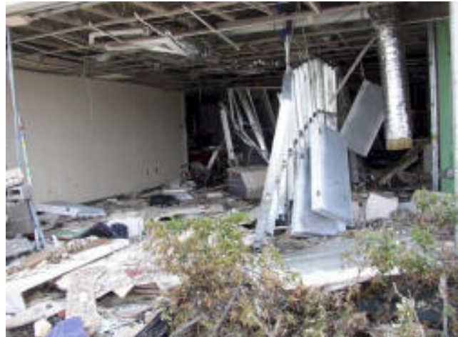
Mississippi Department of Marine Resources- Bolton Bldg.
